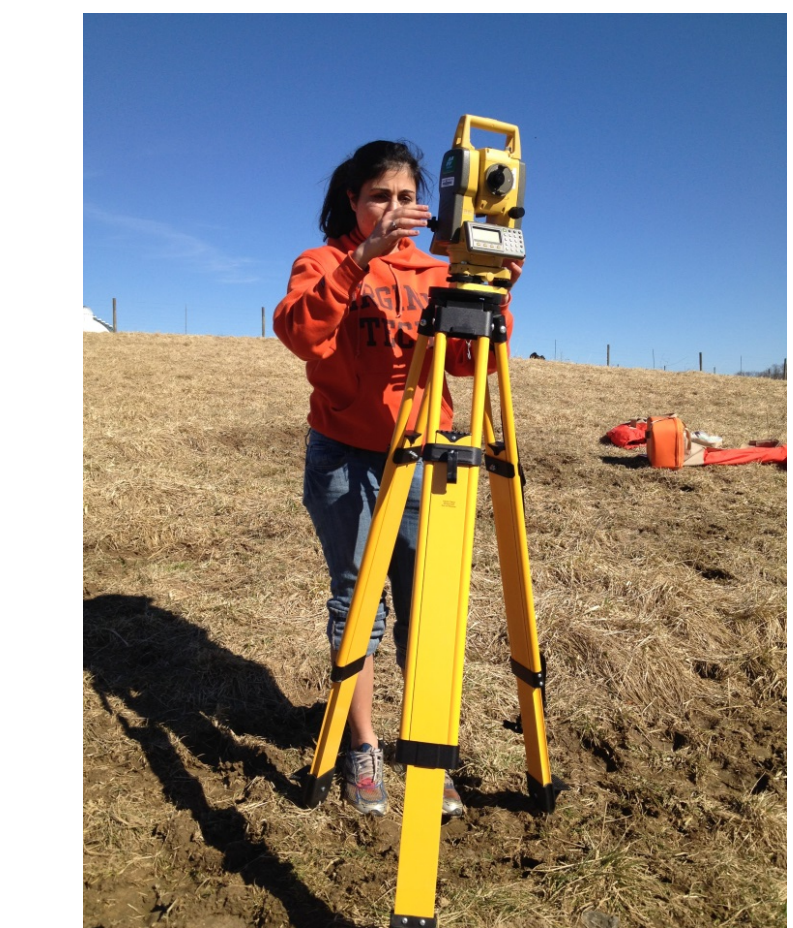
Surveying the site.
