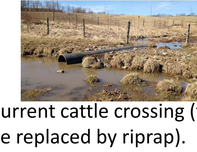
Current cattle crossing (to be replaced by riprap).
